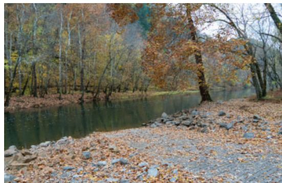
Tailwater Boat Ramp ‘put in’ located below Green River Lake Dam
